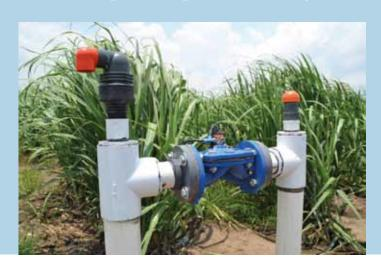
The air valves play a major role in ensuring efficient and reliable operation of the irrigation system.
